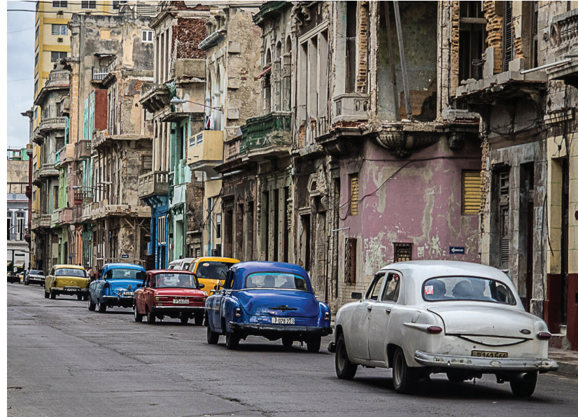
A typical street scene in Havana, Cuba, with its decayed buildings and ever-present antique cars, exhibits the effects of nearly six decades of enforced socialist policies.
